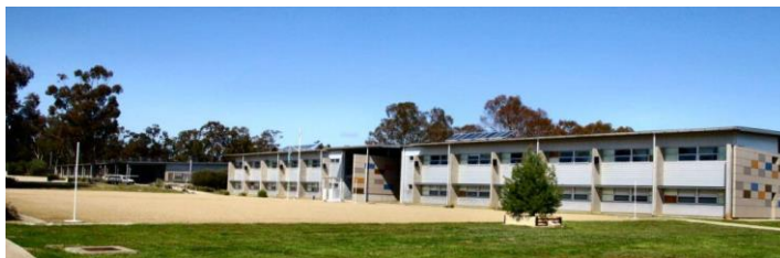
1RTU Living in accommodation
